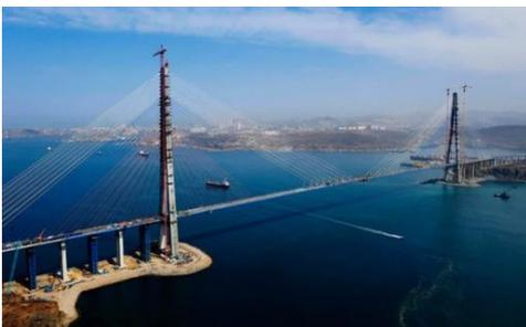
This type of bridge has its roots back in the 16<sup>th</sup> Century. This type of bridge uses cables that are connected to pylons. Usually, the pylons are found in the center of the bridge and other key support areas. These bridges are made to span long **14** \_\_\_\_\_ (**distant**). They can be made out of any material.
