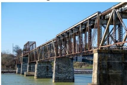
There are many types of truss designs that can be used for construction. One of the most interesting construction types is Pratt. This type of design was used 9 \_\_\_\_\_ (**extensive**) during World War II. The creator of this design was Thomas Willis Pratt and his father Caleb Pratt. This bridge design can span large distances and is easily set up.
